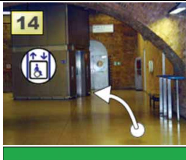
The lift to the Jubilee Line platform is to the left of the ticket barriers .
